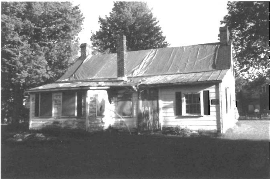
North Elevation, northwest perspective. Lean-to addition (c. 1910) with raised-seam metal roof; green asphalt shingles on log portion; west chimney on right, east chimney on left, north chimney at north wall.
